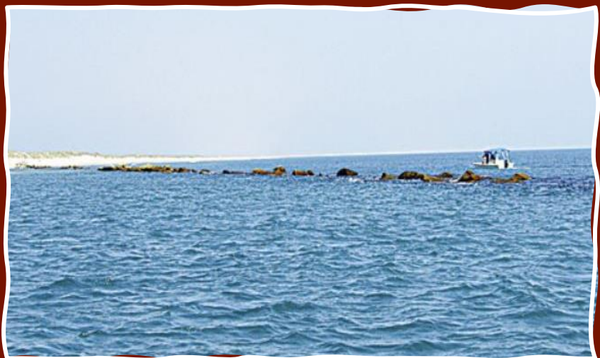
Cape Lookout Rock Jetty picture from https://www.carolinasportsman.com/content/saltwater-series-harkers-island/
